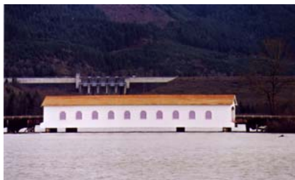
Lowell Covered Bridge is one of three out-of-service covered bridges maintained by the Lane County Parks Division.
