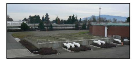
**Description:** Installation of a fourth digester for expanded production of Class B biosolids. This
