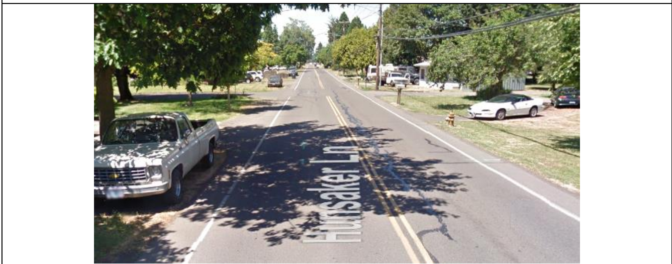
Figure 15. Hunsaker Lane (looking west)
