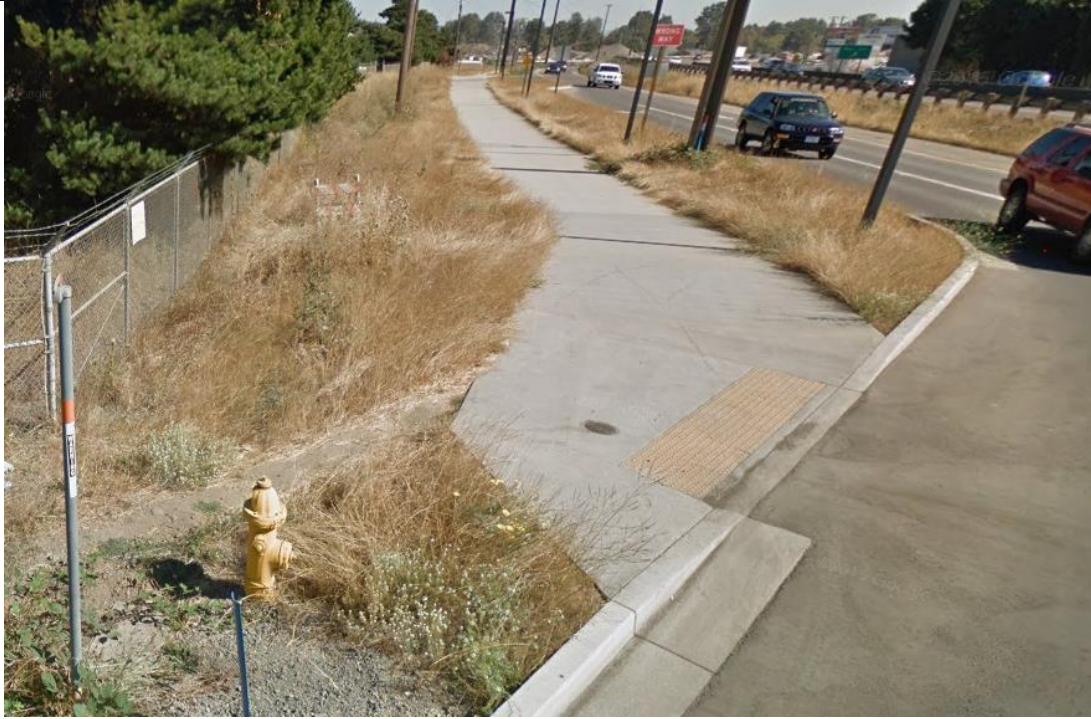
Figure 17. Multi-Use Path (looking east at Division Avenue & Beaver Street)
