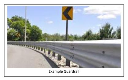
a roadside obstacle as well and have been ranked as a high source of injury and fatal collisions. Engineers must weigh whether placing guardrail will reduce the severity of an impact as compared to what may be impacted if the guardrail were not in place.
