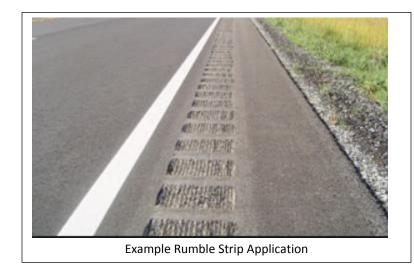
collisions in Lane County. Rumble strips are effective (and cost-effective) at reducing collisions due to inattention.
